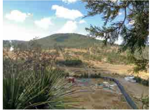
Looking at part of the geothermal plants in Los Humeros (Photo: A. Jentsch, GFZ)
