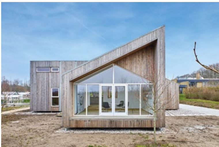
World's first house from waste and scrap materials from the agricultural industry. It is exhibited at the BIOTOPE ecological park in Middelfart, Denmark
