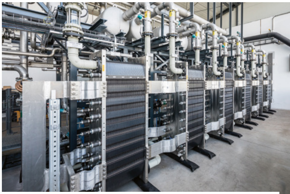
Installation and Operation of an Electrolysis System at the Steel Production Site in Linz, Austria
